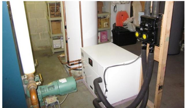
Bosch TW035 water-to-water system provides domestic hot water
