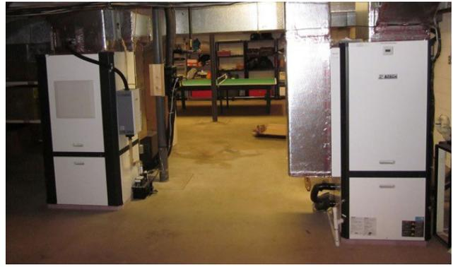
Two of six Bosch SM two-stage geothermal heat pumps installed in basement
