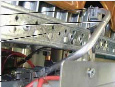
3. Remove lower end of pilot tube from black clip on gas valve being careful not to damage cylindrical air screen
