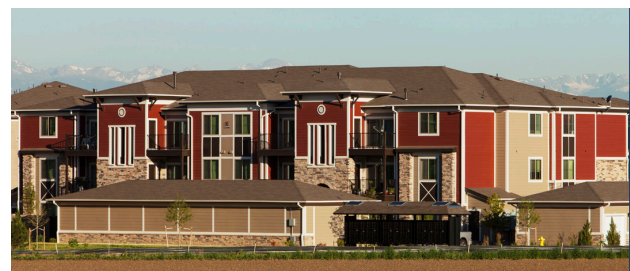
Solaire Apartment complex
