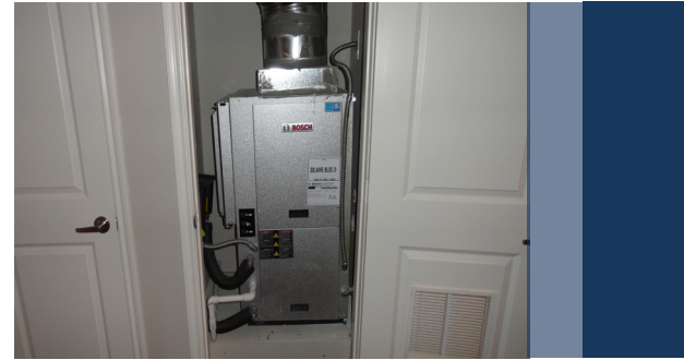
252 Bosch BP Series water-to-air geothermal heat pumps can provide 326 tons of heating and cooling to serve all the apartments
